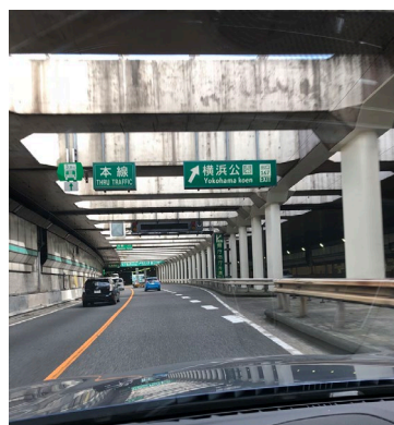
Fig.12 Completed open-cut motorway near Yoshida canal. Source: own elaboration.
