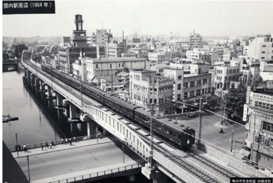
Fig.7 Haohka canal viewing Kannai district on the right. Photo courtesy of the City of Yokohama.
