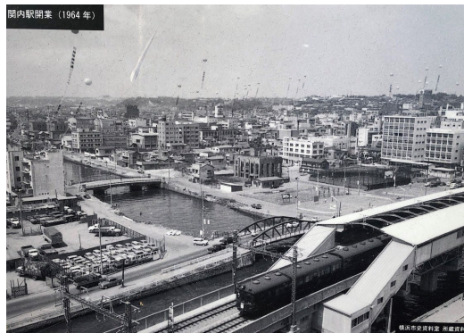
Fig.8 Yoshida canal viewing inland areas towards the south-west. Photo courtesy of the City of Yokohama.
