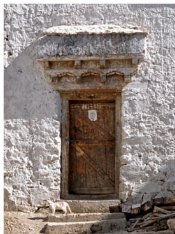
Top Left: Typical Ladakhi windows and balconies Top Right: Entrance to an ordinary house in Leh with typical Tibetan lintel Below: An ordinary house in Leh showing stone masonry at lower level and adobe bricks at upper level
