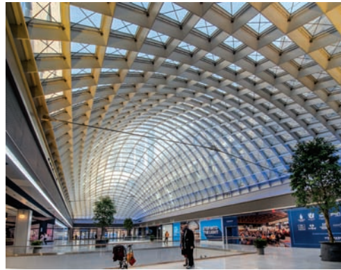
Left: Step into the light - one of several day-lit courtyards of Moynihan Train Hall Bottom: A new gateway to the city: The conversion of the old mail sorting room into a light filled concourse. The design retains three existing steel trusses and adds a newly engineered vaulted glass roof that allows daylight to fill passenger spaces and create a contemporary public space
